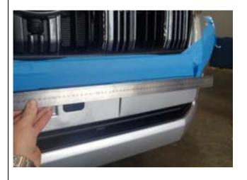
8. Using a straight edge, rule a horizontal line across the front of the factory bumper 30mm above the top edge of the number plate recess.
