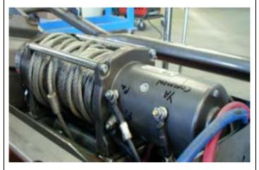
14 With the roller fair lead previously in position, lift the winch into position and bolt into place using the 3/8" hardware supplied with the winch, bolt securely in place.
