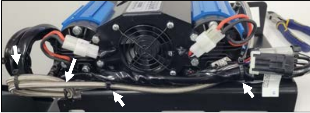
Figure 8. Retention of air line and harness with cable ties
